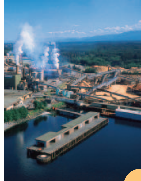
Figure 4.6 Pulp mill in British Columbia
