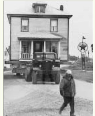
Figure 4.11 In the 1950s, a series of dams was built on the St. Lawrence River. The reservoir that was formed left the sites of six villages underwater. The above photo shows a house being moved away from the area about to be flooded.
