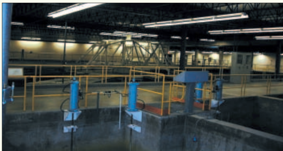
Figure 4.16 By monitoring water throughout the year, technicians in this water treatment plant know when they have to add more chlorine.
