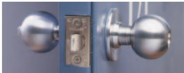
Figure 1.12 A doorknob is a wheel-and-axle machine. Which part is the wheel and which part is the axle?
