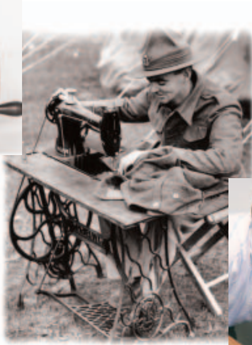
Figure 3.14a) Early sewing machines were operated by a hand crank. They could sew only simple stitches.
