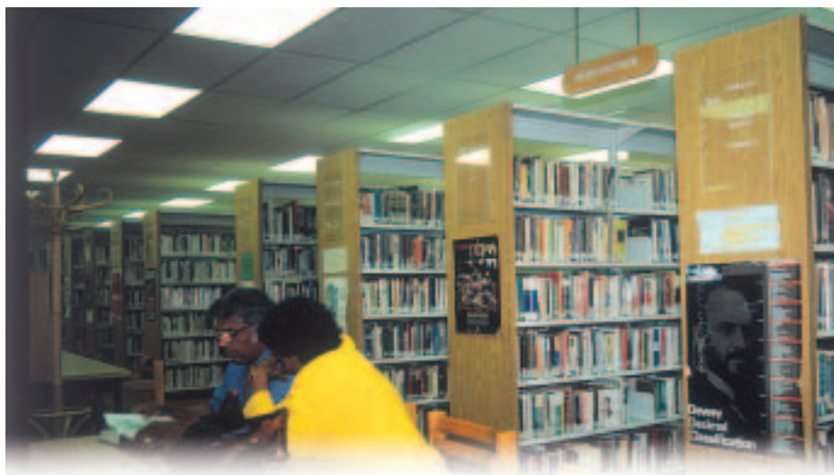
Figure 3.14 Fluorescent lights are commonly used in offices and public buildings.
