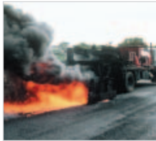
Figure 3.2b) Hot tar spread on a road
